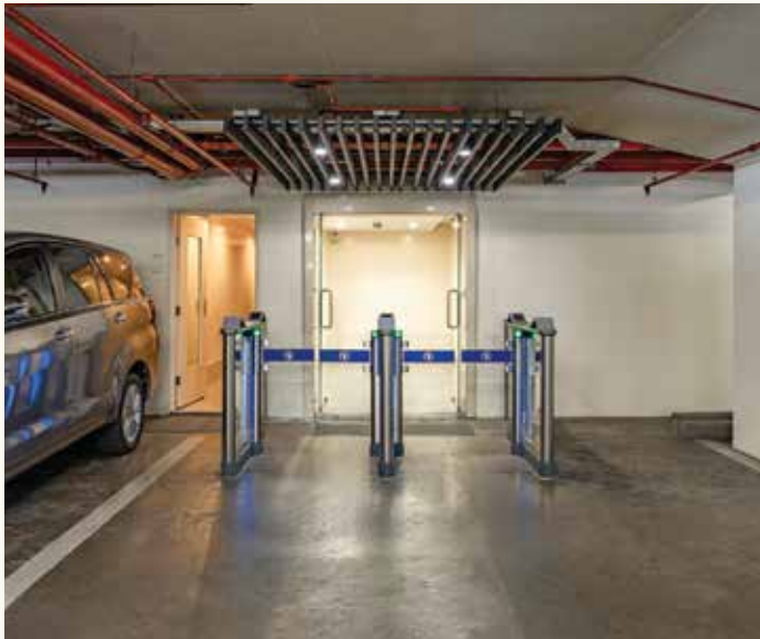
Turnstile & Lobby in Basement
